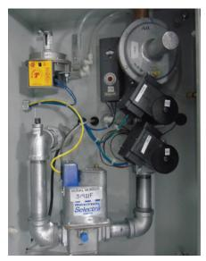
Gas controls allow either natural or LP gas, and higher gas pressures allow greater heat output.
