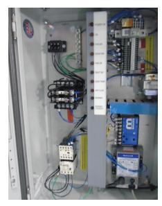
Advanced electrical controls include an airflow switch and temperature stat.
