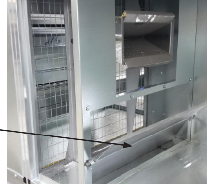
Automatic Burner Profile Damper
