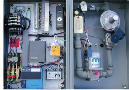
Reliability is ensured with advanced gas-manifold controls, electronic ignition, flame rod burner supervision, and diagnostic circuit check lights.
