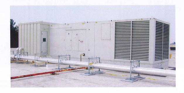
Process loads can vary throughout the day with, for example, intermittent paint booth operations or welding processes. Direct gas-fired heating systems allow convenient and flexible control of ventilation rates to match these loads.
