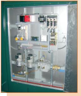
All wiring, piping, and electrical- and gascontrol components are expertly assembled in modules behind sealed, easy-access panels.
