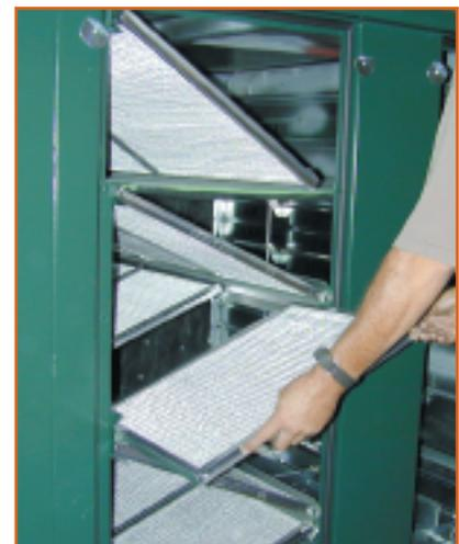
**Cleanable or replaceable filters** for incoming fresh air or recirculated conditioned air are readily accessible for service.
